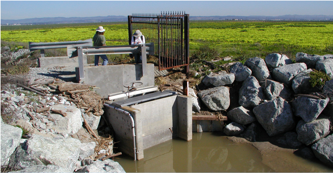
Photo P6.2 Tide gate Photo: ESNERR
