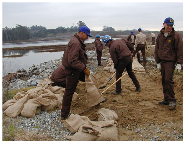
Photo P2.3 Repairing water control levy Photo: ESNERR
