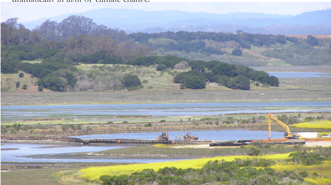
Photo P3.3 Large scale repair on existing water control structure Photo: ESNERR
