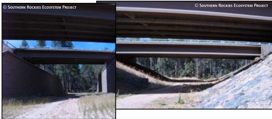
RESEARCHERS AT THE AZ GAME AND FISH DEPARTMENT HAVE SHOWN THAT WILDLIFE PREFER THE SLOPED, MORE NATURAL UNDERPASS (RIGHT) TO HARD-EDGED WALLS (LEFT) ON STATE ROUTE 260.
