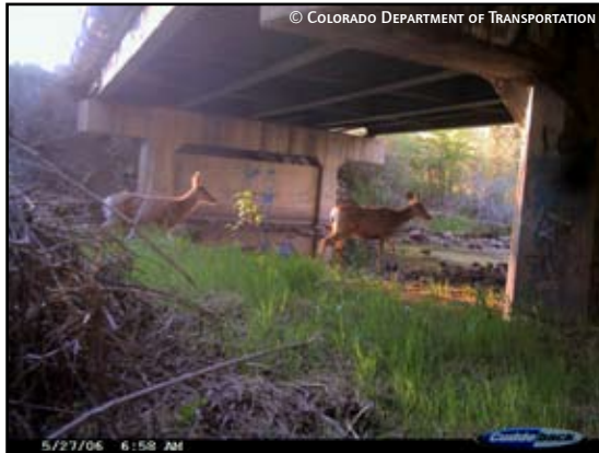
MULE DEER CROSSING UNDER A BRIDGE EXTENSION ON THE FLORIDA RIVER ON US HIGHWAY 160 NEAR DURANGO, COLORADO.
