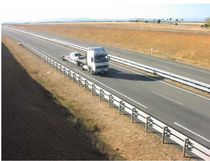
**Figure 41: Metal beam barrier and guardrail.** Photo by A. P. Clevenger.
