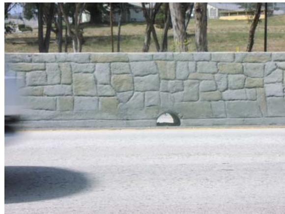
**Figure 1: Caltrans included basal openings in the Highway 1 concrete barrier for small animal passage. Photo by A.P. Clevenger**
