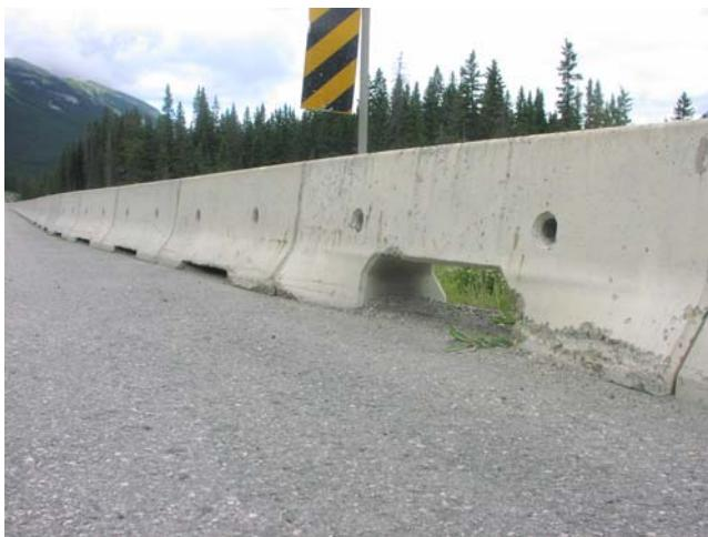
**Figure 40:** Concrete barriers with scuppers for small to mid-sized animal passage. Photo by A. P. Clevenger.
